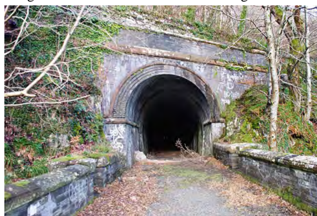
South portal of Tregarth tunnel in January 2013.
